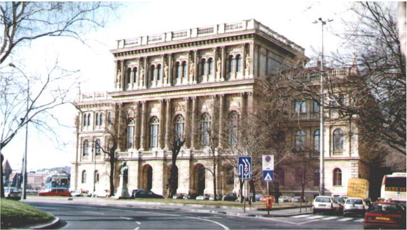
The classical building of the Hungarian Academy of Sciences, the site of the Mid-term Symposium of the Commission VII in Budapest
